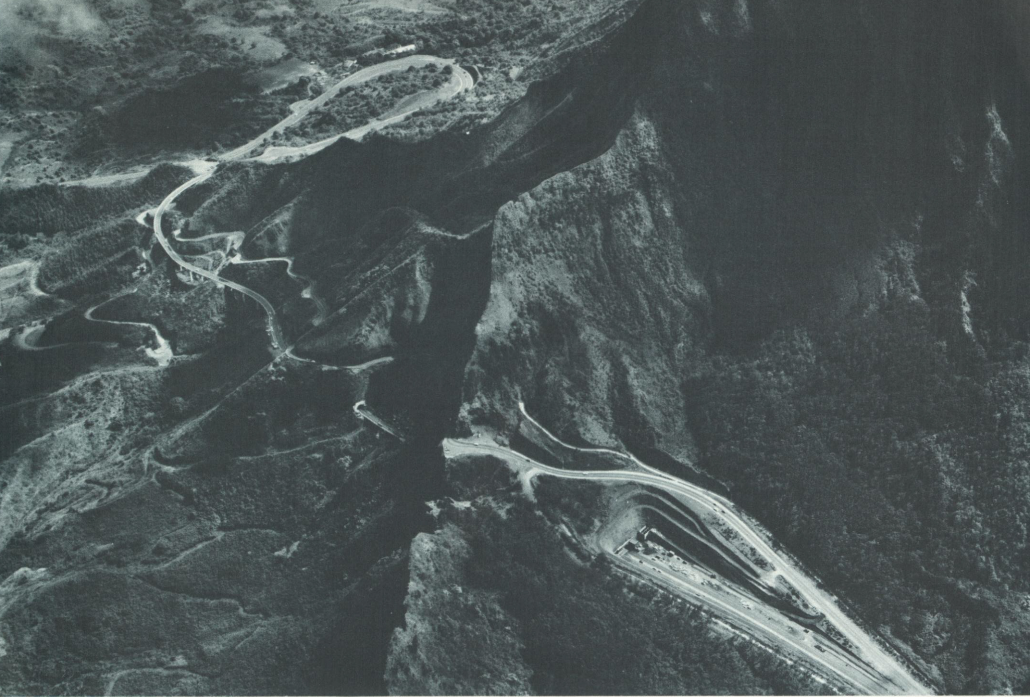
Tunnels and new highways through Koolau Mountain Range at famed Pali peak have speeded traffic from Honolulu to opposite side of Oahu and aided phenomenal growth there. Resulting new load demand has spurred construction of the Islands' first 138 kv lines from Waiau Plant over ridge to Windward Oahu
