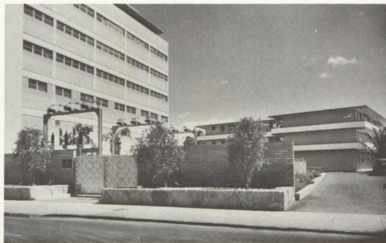
Five new substations were installed during 1959. All were planned to blend into surroundings. Landscaped Waikiki substation above is typical.
