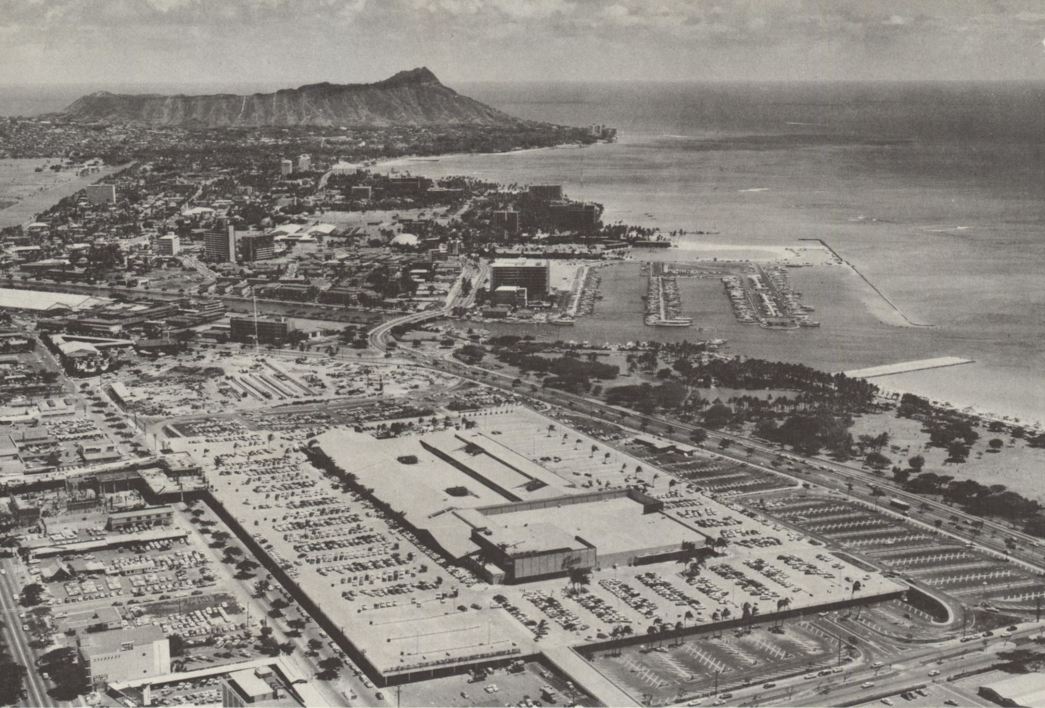
Ala Moana Center, foreground, is an emphatic sign of Honolulu's economic growth in 1959. Huge shopping area, one of nations 10 largest, is at gateway to Waikiki, where new hotels and apartments are fast changing the skyline stretching to Diamond Head. Center's 80 stores demand 6,000 kilowatts of power every day.
