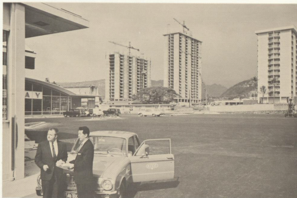
The $10.2 million Queen Emma Gardens in downtown Honolulu, shown nearing completion, features 582 apartments with all-electric kitchens. In foreground is shopping center developed to serve the area. Commercial sales representative assists N. C. Adams, district manager of Long's Drug Stores in Hawaii.
