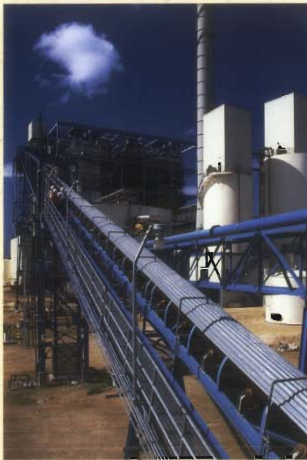
Low-sulfur coal to power generators will be carried up the long conveyor at the 180-megawatt plant owned by AES Barbers Point, Inc. HECO will purchase the power when the plant at Campbell Industrial Park west of Honolulu is completed in late 1992.
