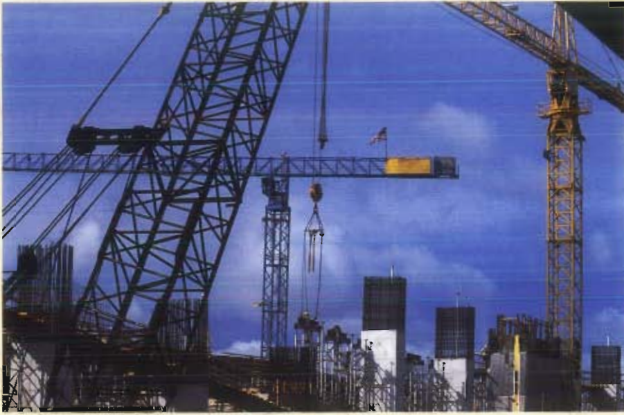
Cranes and reinforced concrete form a lattice at the new interisland terminal and parking facility under construction at Honolulu International Airport. Completion is planned for 1994 and will add 13 gates and parking for 1,800 vehicles.
