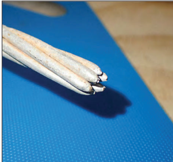
Figure 54: Image of FCA Artifact DB#29, B-Phase dead-end conductor attached to Pole 25 that did not exhibit melting and appeared to have experienced tensile failure
