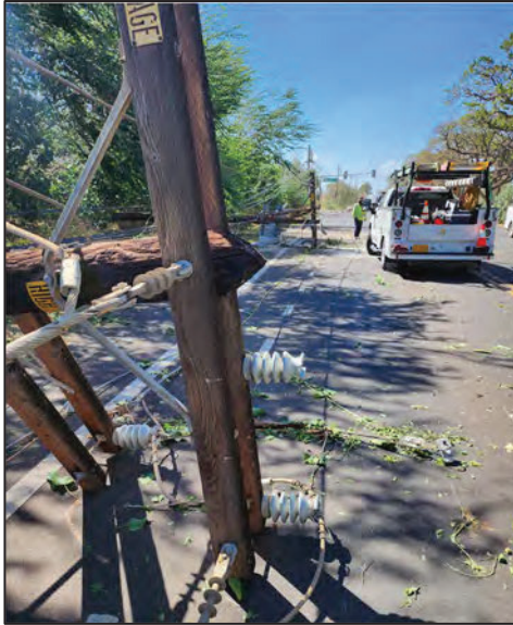
Figure 18: Photo captured by a Hawaiian Electric substation engineer at 9:25 a.m. of a series of poles across Honoapiilani Highway near the intersection with Hokiokio Place
