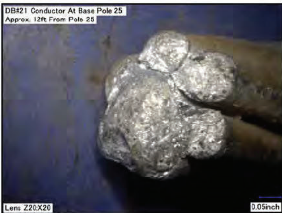
Figure 52: Microscope image of FCA Artifact DB#21, C-Phase dead-end conductor attached to Pole 25 that exhibited melting associated with phase-to-phase fault current
