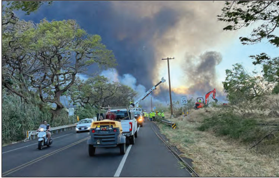
Figure 36: 6:11 p.m. north-facing photo captured by a contractor showing traffic moving southbound while contractors work in the northbound lane of Honoapiilani Highway
