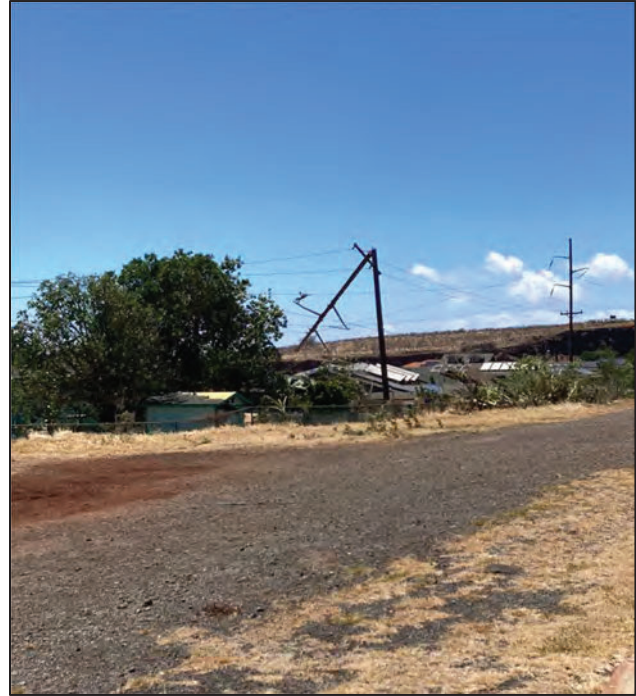
Figure 22: 2:10 p.m. photo captured by a Hawaiian Electric foreman of Pole 9 on Niheu Place leaning into the backyard of a residence
