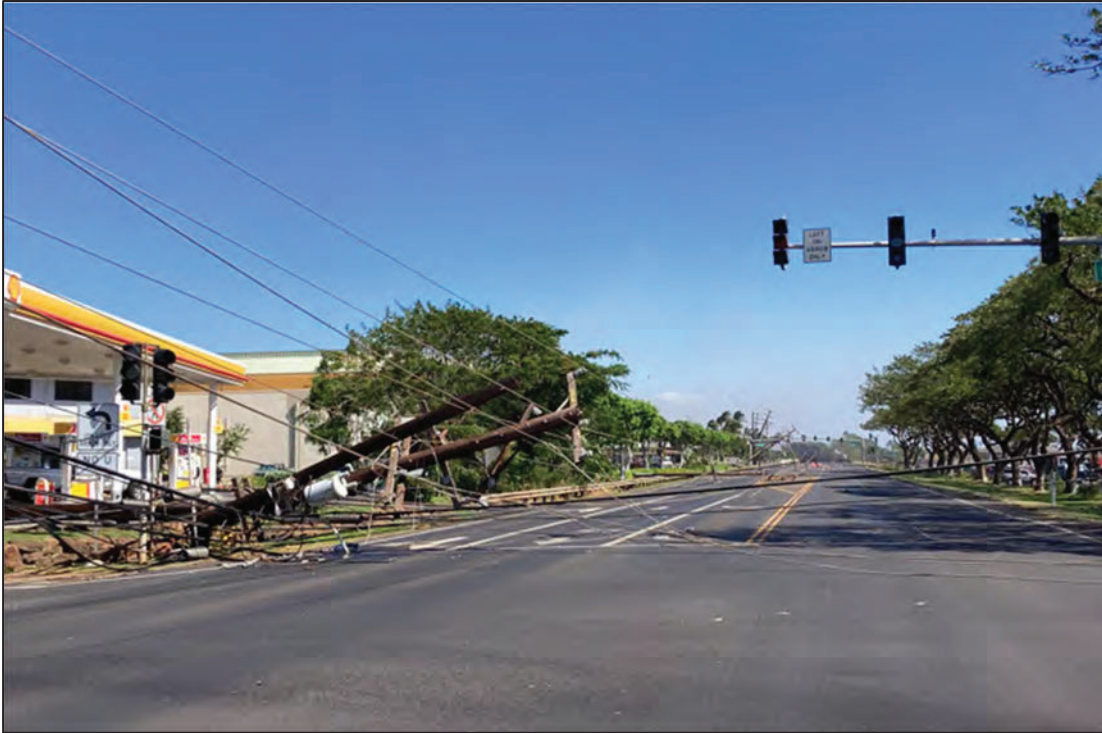
Figure 39: Photo by a Hawaiian Electric Troublemaker from approximately 3:22 p.m. of additional poles down at the intersection of Honoapiilani Highway and Kapunakea Street (exact metadata not available) that could be bypassed via the Safeway parking lot
