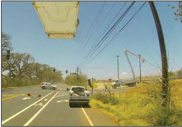
Figure 31: 12:59 p.m. north-facing dashcam photo captured by a contractor showing poles down across Honoapiilani Highway and a MPD cruiser stopping traffic at Hokiokio Place
