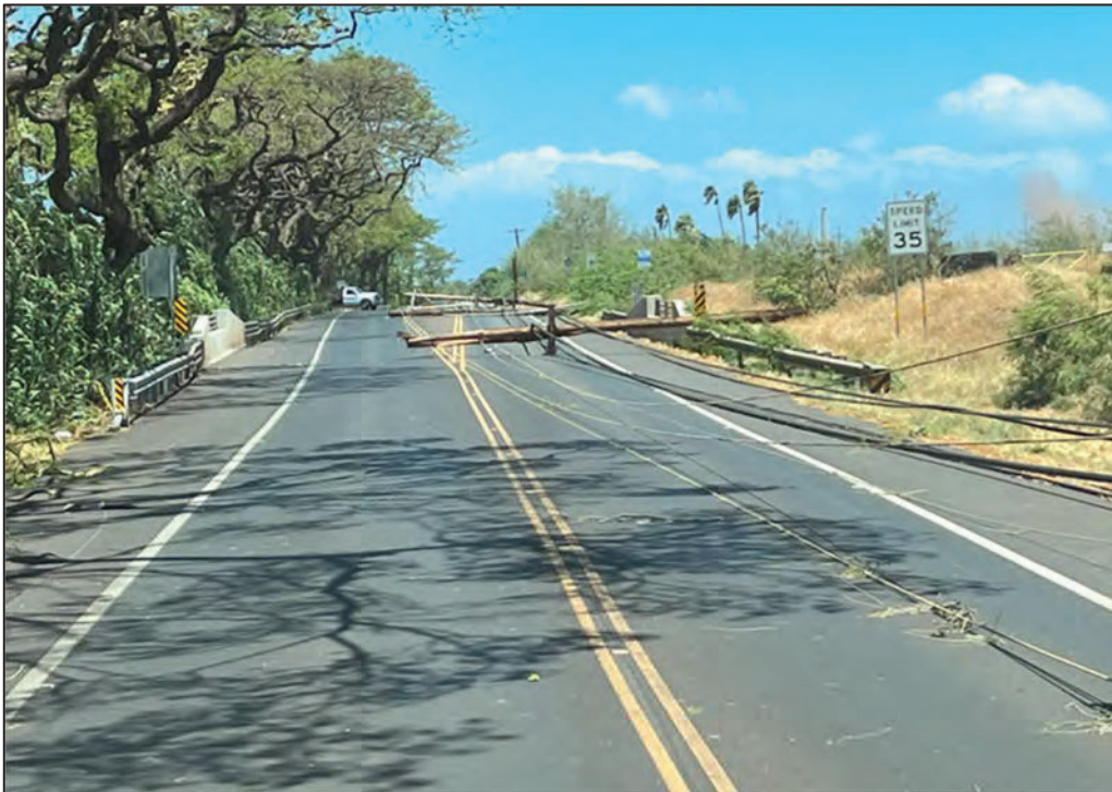
Figure 20: Photo captured at 11:40 a.m. by a Hawaiian Electric foreman of lines and poles down on Honoapiilani Highway
