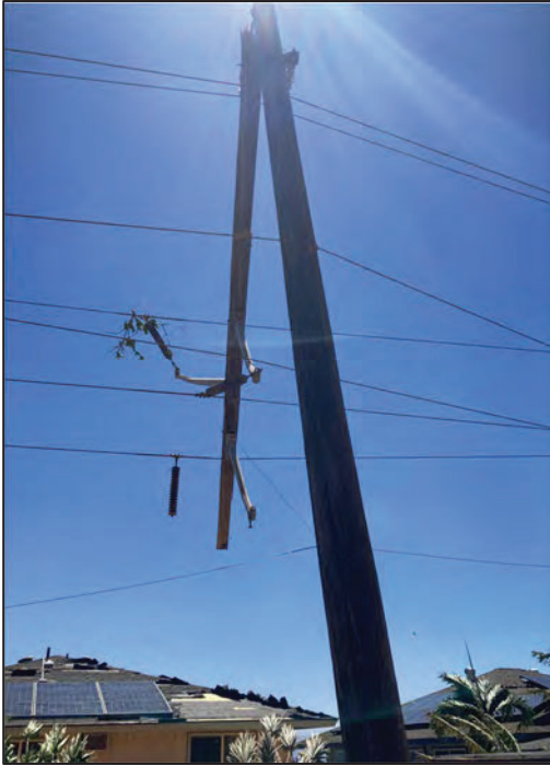
Figure 21: 2:18 p.m. photo captured by a Hawaiian Electric foreman of Pole 9 on Niheu Place leaning into the backyard of a residence
